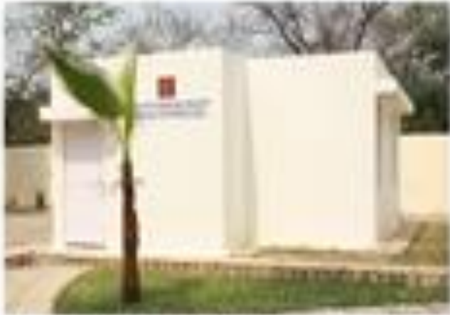
EPS with Double Panel & RCC
