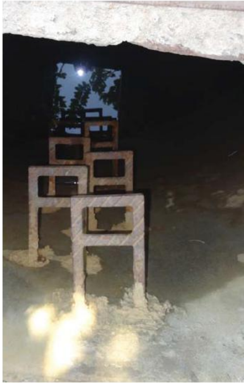
UNCOVERED WATER TANK
